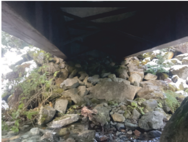
Left Bank Abutment when facing downstream
