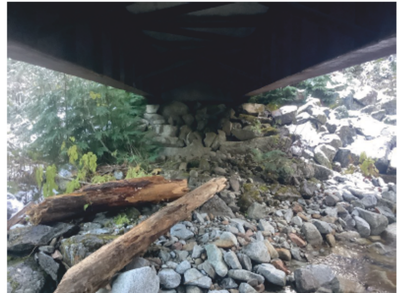
Right Bank Abutment when facing downstream
